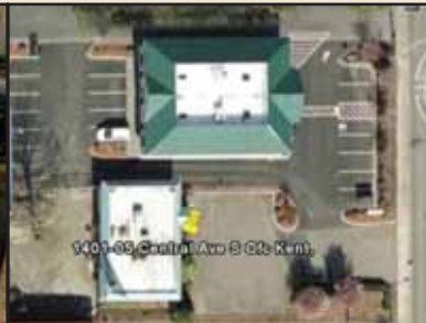
1,950 SQ. FT. OFFICE BLDG. AND 3,850 SQ. FT. RETAIL BLDG.
