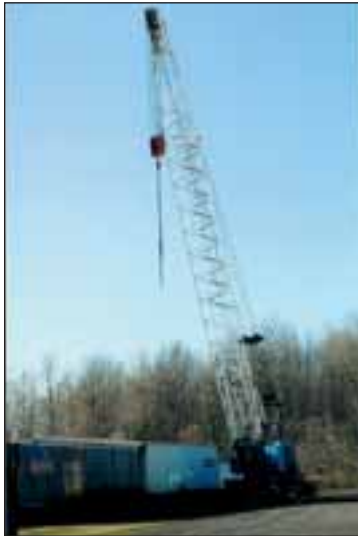
P&H 9125-TC 140 Ton Capacity Truck Crane
