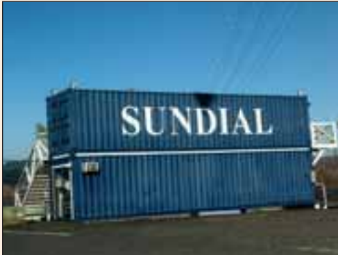
(2) 40' Double Stacked Containers Converted to Locker Rooms
